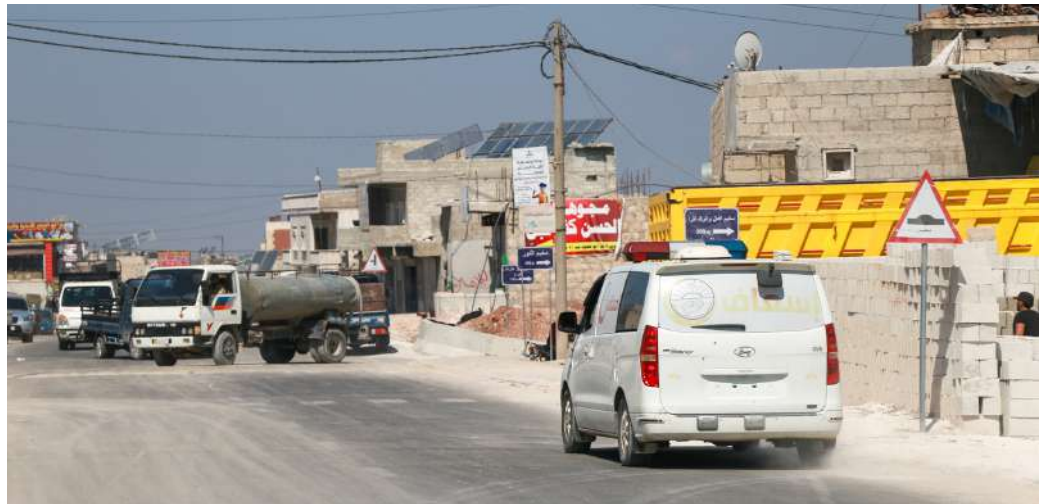
Figure 13: The recently repaired Qat-Atmeh road (Photo credit: BINAA)
